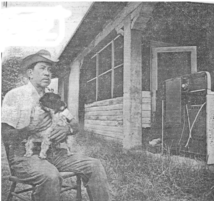
John V. Callahan sits outside the adobe almost completely constructed from parts of the main house. It was dismantled in 1909.
