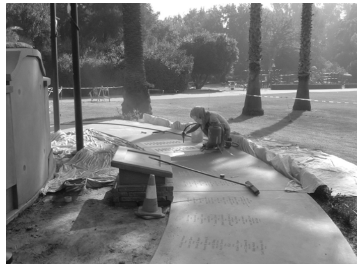
Sandblasting names in concrete from the Veterans Walk
